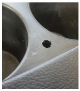
6. With the panel in place, pre-drill 4x holes using a 3.2mm (1/8") bit
